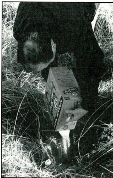
After digging a hole and pounding in a copper pipe, Guy Atkins fills the hole with clay clumping cat litter.
