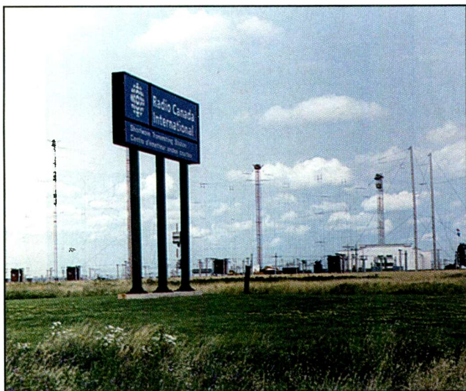
The clear, strong signals from Radio Sweden and Voice of Vietnam are thanks to these broadcasters being relayed by the RCI site at Sackville, New Brunswick.
